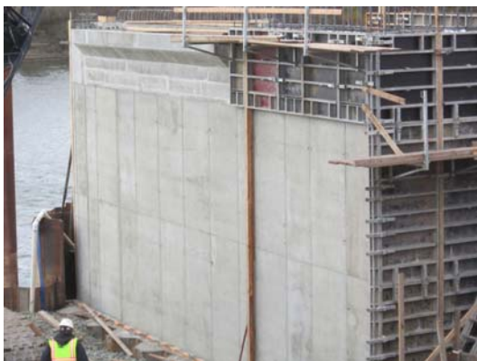
Diversion facility south wall
