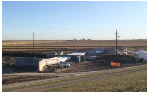
Completed NDC Structures and 72-inch WSP
